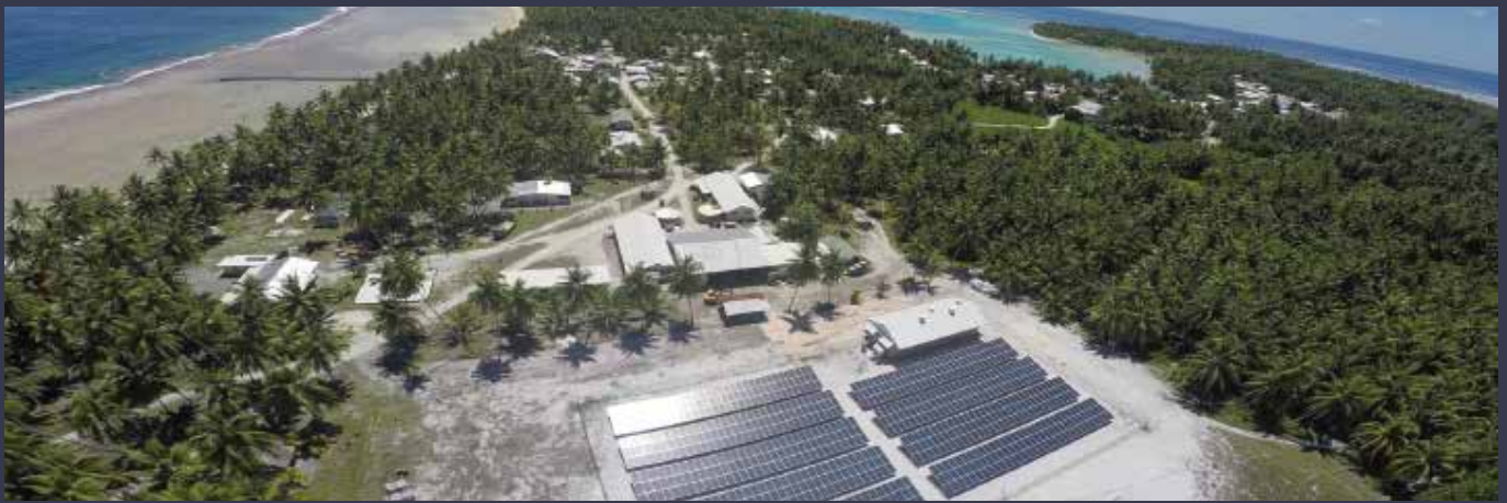
Pukapuka Solar-diesel Hybrid Community Power Station, Cook Islands
